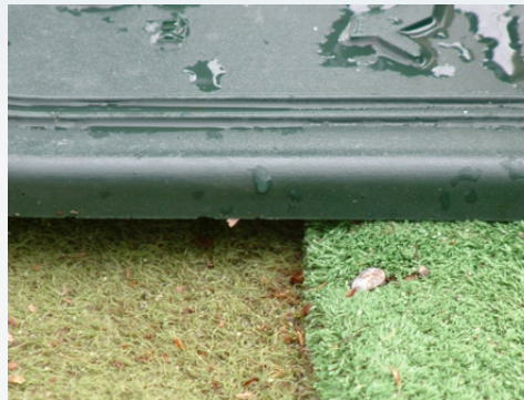
Unsatisfactory joining of surfaces.
