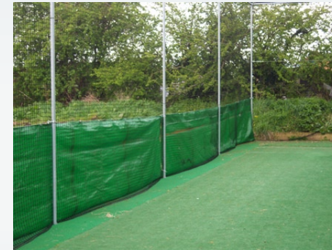
A rodent protection skirt on the outside of the net.
