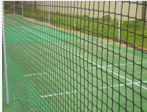
Tension wire ready for fastening to the net to reduce billowing.
