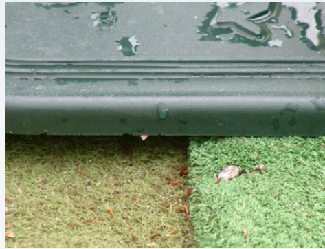
Unsatisfactory joining of surfaces.
