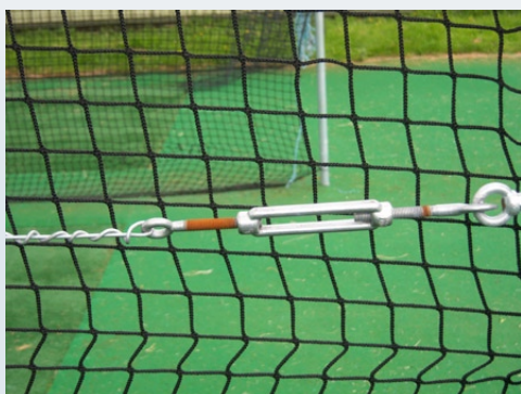
Fixing holding the tension wire for reducing billowing.
