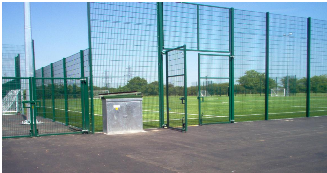
Gates should open outwards – double gates should be provided for access by maintenance plant and emergency vehicle
