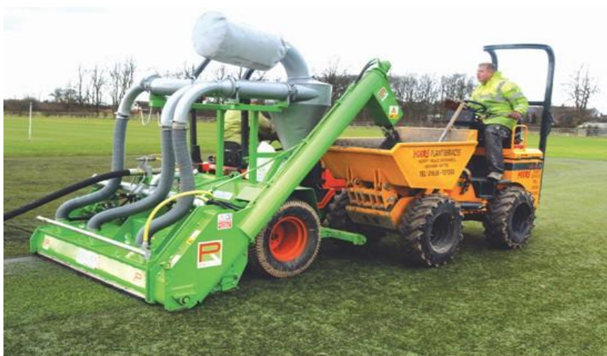
Replacement of contaminated infill
